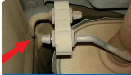
Exhaust hanger contacting the frame hanger.
