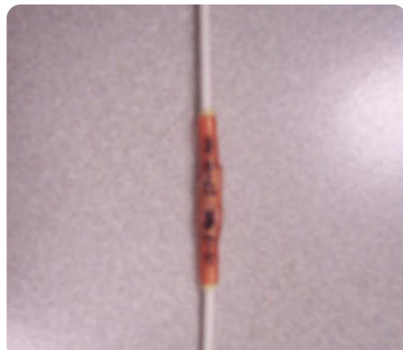
Wire spliced and sealed with heat shrink tubing
